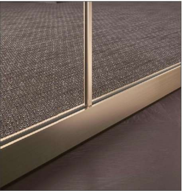
I-profile connection for straight glass joint
